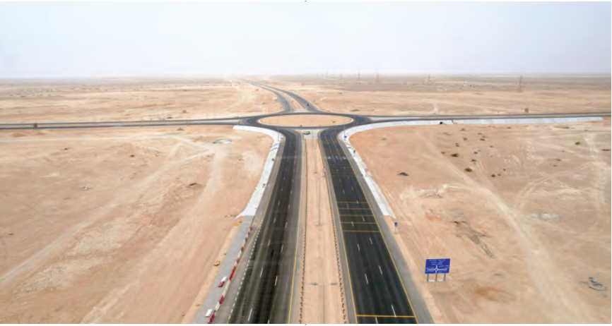
The project is intended to improve access within the SEZAD.
