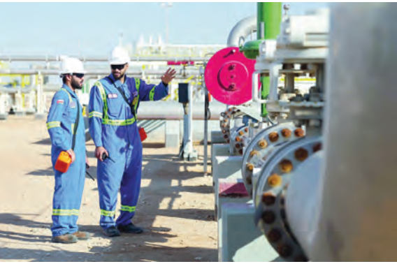
PDO recorded 555 electrical incidents and protection events during the period, with approximately half resolved remotely.
