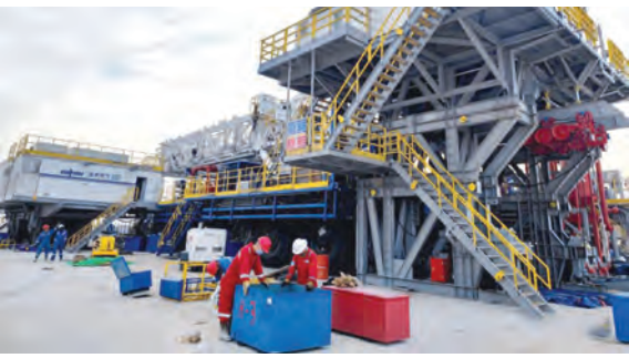
A BOMCO automated drilling rig in Oman.
