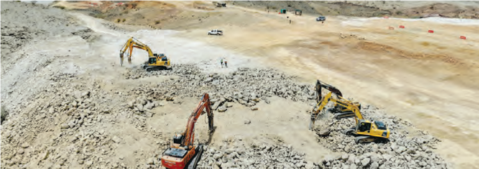
The project involves the construction of a 7-kilometre-long, 900-millimetre-diameter water pipeline to transport water from the dam to the purification plant.
