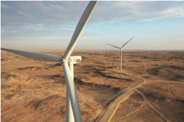
Construction officially commenced in June 2026, with commercial operations targeted for Q3 of 2027.
