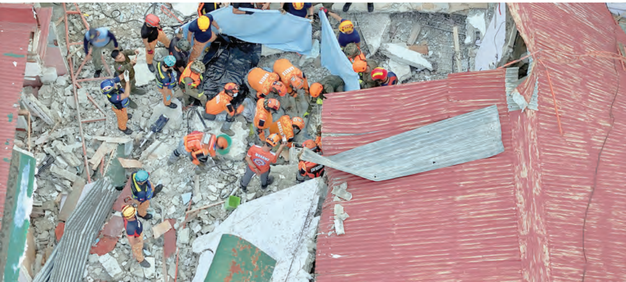
A drone view shows rescue workers conducting a rescue operation in Bogo, Cebu, Philippines. — Reuters
