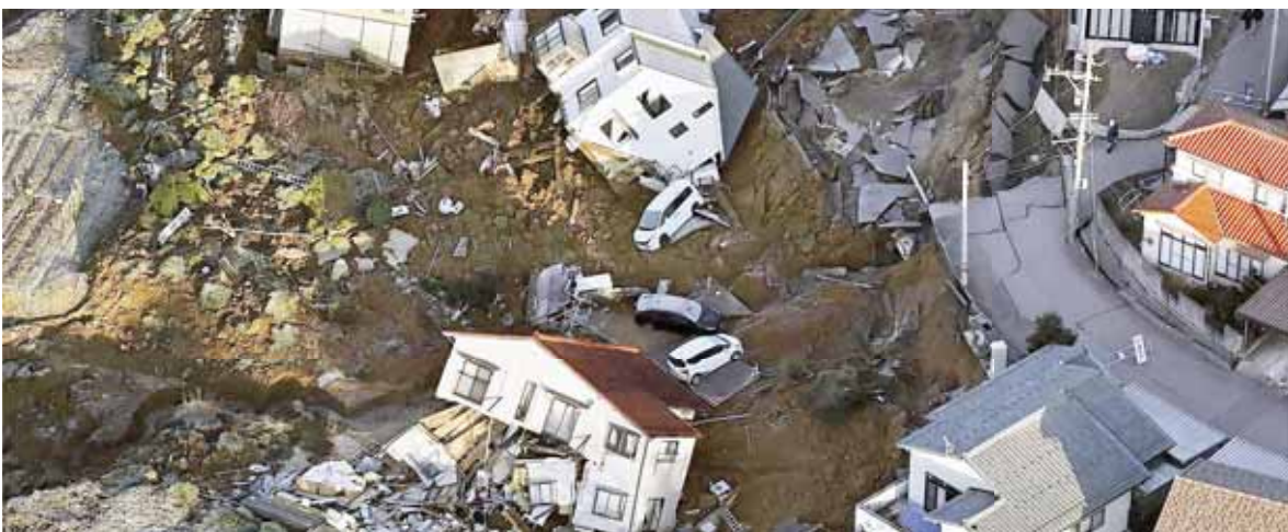
Destoryed houses in Kanazawa, Japan
