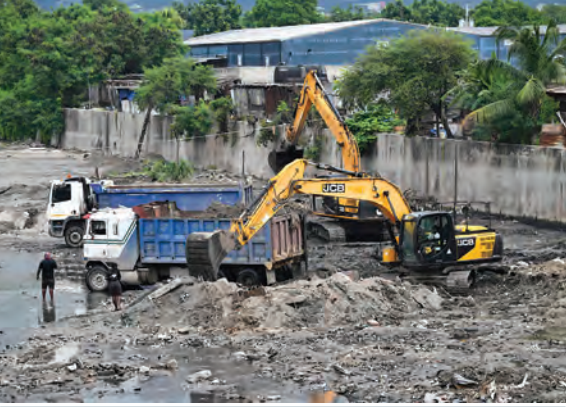
Crews clean the main diversion channel for floodwaters in preparation for the arrival of Hurricane Melissa, in Kingston, Jamaica. — AFP
