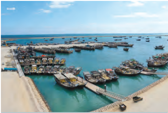
The project will include roads, lighting, drainage, sewage, water and communication networks.
